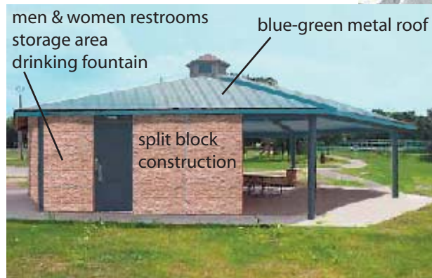
Partially enclosed HXE 48 TG Polygon framing and roofing
