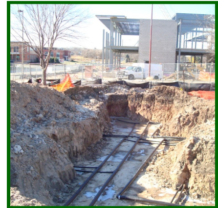
Geothermal heat exchange system construction.
