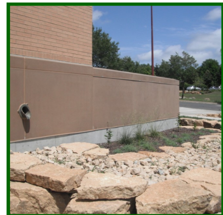
Stormwater is kept on-site as much as possible.
