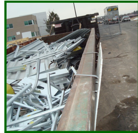
Construction recycling container for collecting metals .
