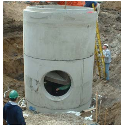
Below-Ground Storage Device
