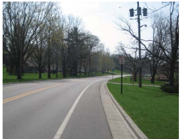
Ski Lane has Bicycle Lanes but no Sidewalks
