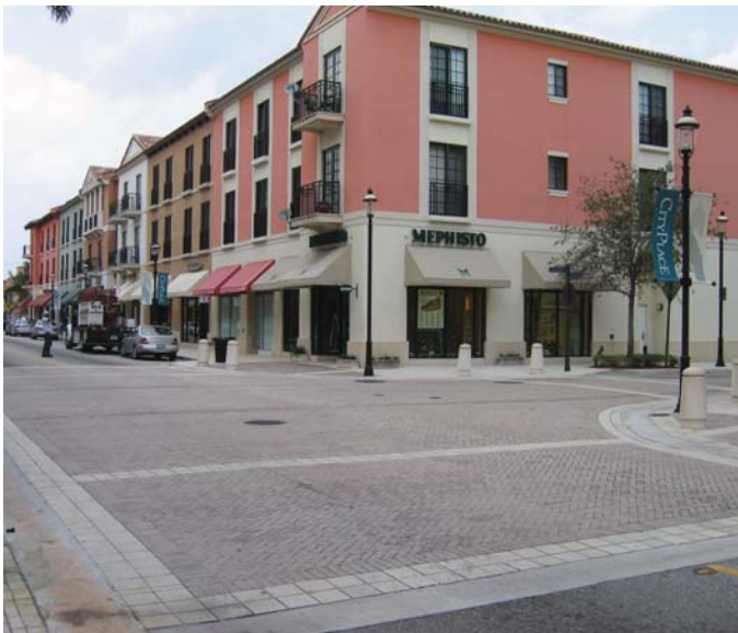
A raised intersection puts crossing pedestrians at a higher, more visible level.
