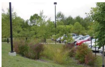
Filtration/ Infiltration through a Bio-Swale
