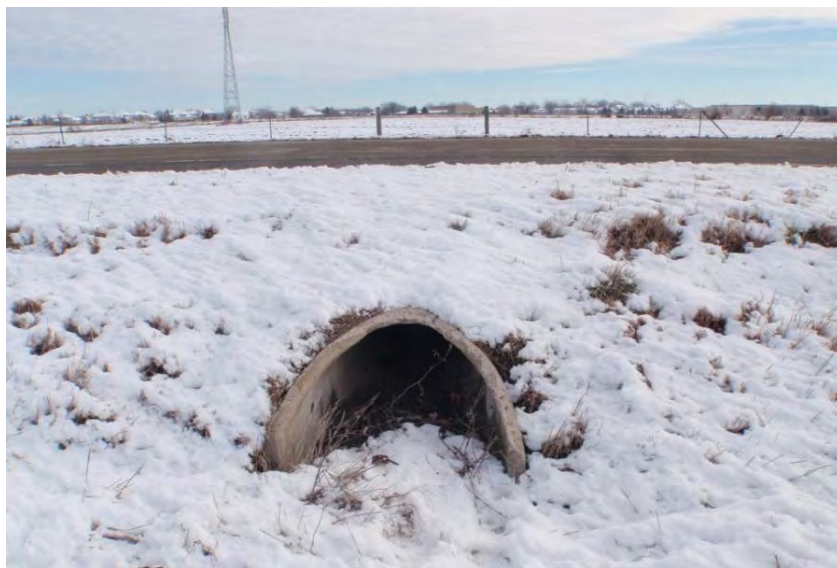
Figure 6-5. 18-inch culvert under Seminole Highway approximately 1700 feet north of Lacy Road.
