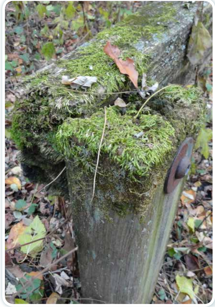
Figure 33. Dilapidated timbers of parcourse equipment
